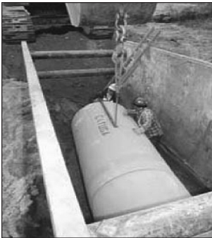
These workers are protected from a cave in and have safe access and egress from the trench.
