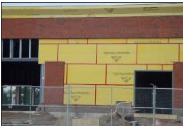
Photo of rigid air barrier
