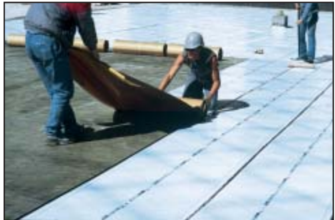
Rolled, self-adhering waterproofing membrane (MEL-ROL)
