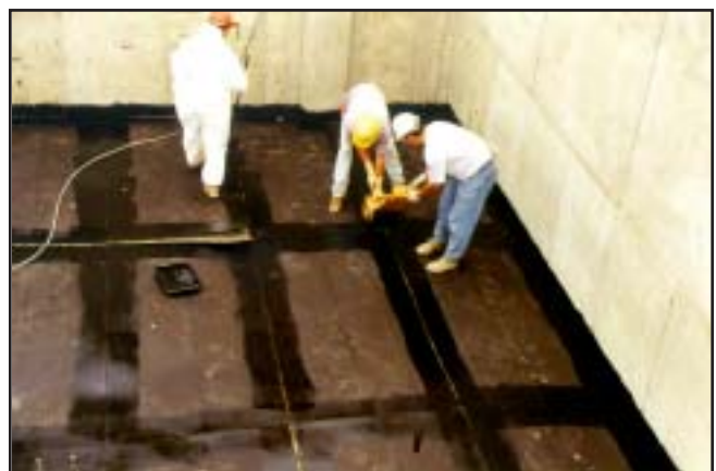
Detailing joints of ASTM E-96 vapor barrier (PREMOULDED MEMBRANE VAPOR SEAL with PLASMATIC® CORE)
