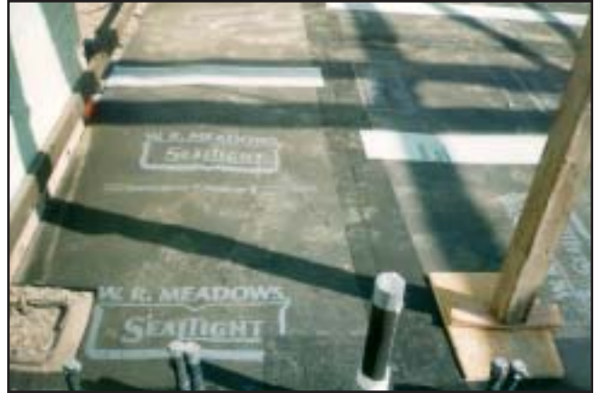
Application of ASTM E-96 vapor barrier (PREMOULDED MEMBRANE® VAPOR SEAL with PLASMATIC® CORE)
