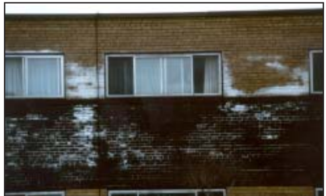
Photo of efflorescence. Photo supplied courtesy of Retro-Specs Consultants, Ltd. (Kevin Knight)
