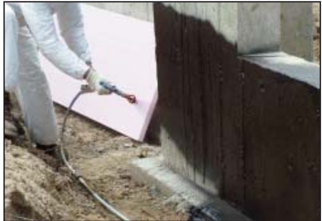
Spray-applied waterproofing membrane (MEL-ROL LM)
