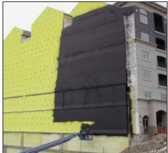
Liquid-applied vapor permeable air barrier (AIR-SHIELD LMP).
