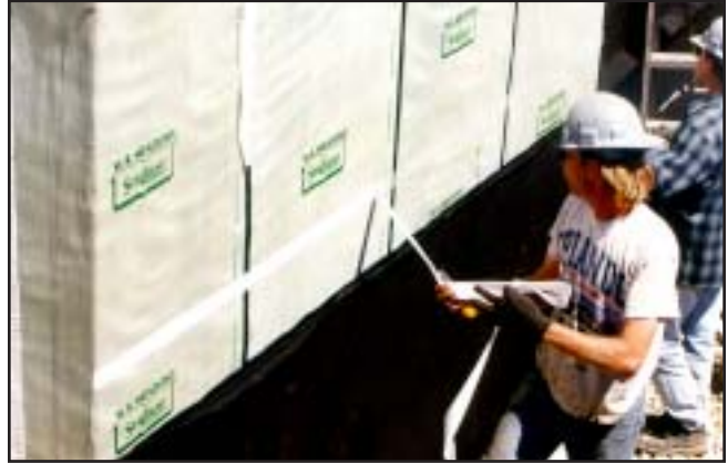
Sheet-applied waterproofing membrane and drainage layer (MEL-ROL® Waterproofing Membrane and MEL-DRAIN™ Drainage Board)
