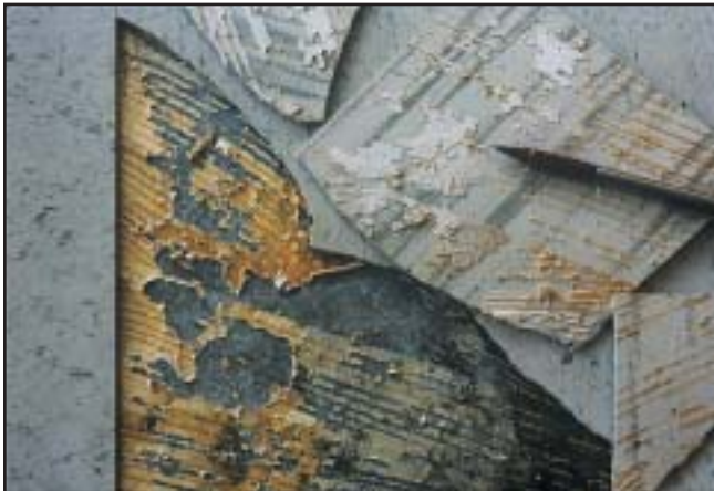
Photo courtesy of Mr. Robert Cox, Construction Consultant
