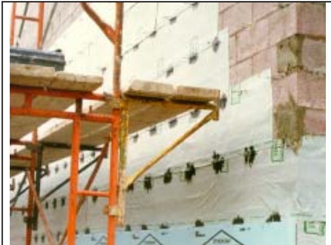
Flexible sheet-type membrane air barrier being applied to exterior wall. (AIR-SHIELD)
